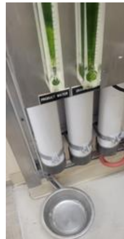
Algae contamination in a Reverse-Osmosis System Rotameter
