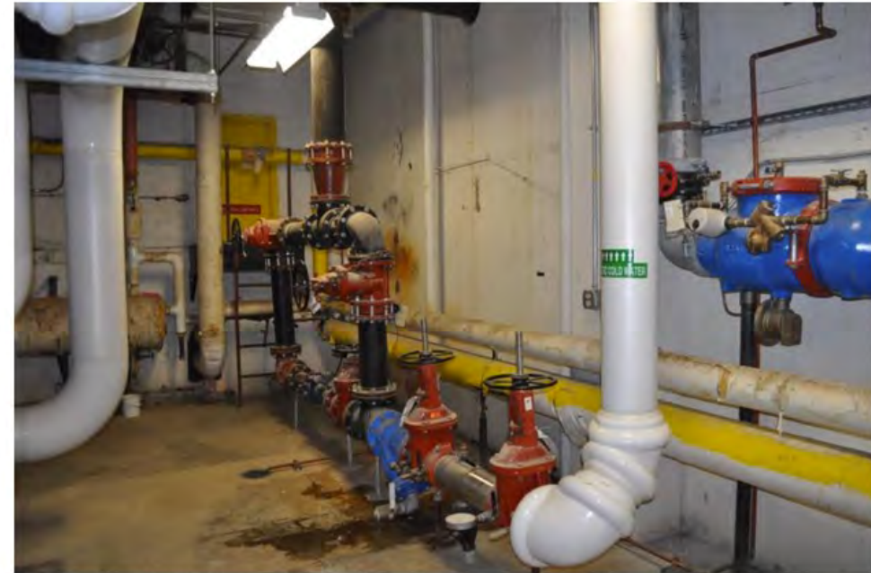
Fig 1. Building Containment - protects upstream public water supply from building domestic water and fire protection water (Not Organization Facility).
