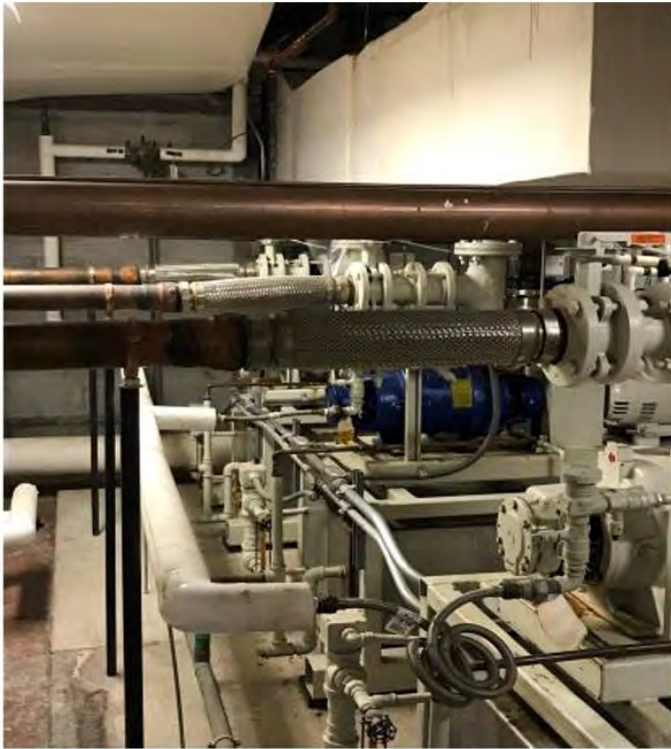
RPBP in Common Supply - Medical Vacuum Pumps.
